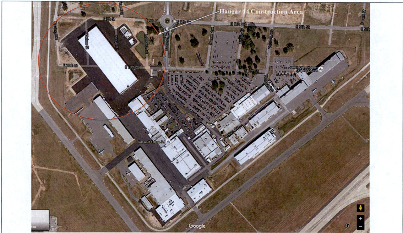
Overall satellite image showing completed Hangar 14 and surrounding pavement.
