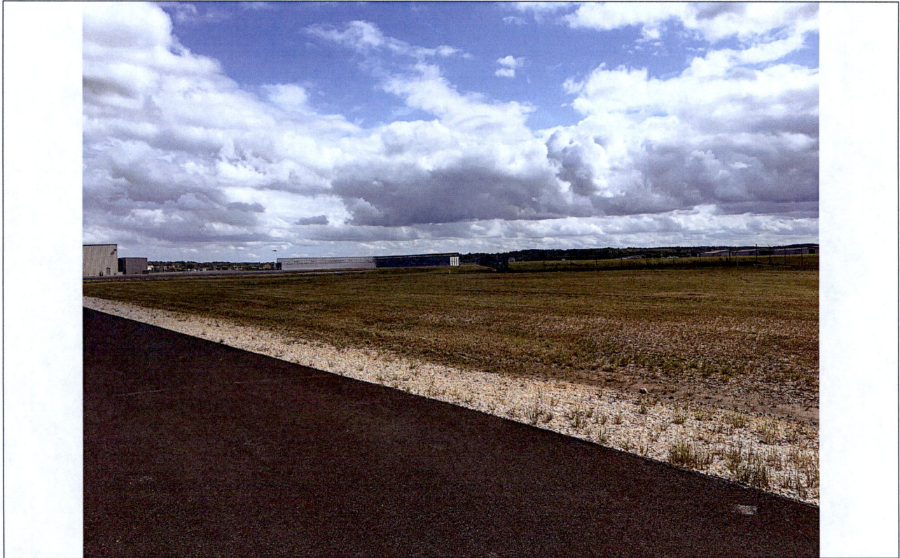
Area around Stormwater Detention Pond on west side of Hangar 14.
