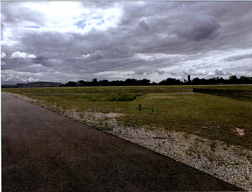
Area around Stormwater Detention Pond on north side of Hangar 14.
