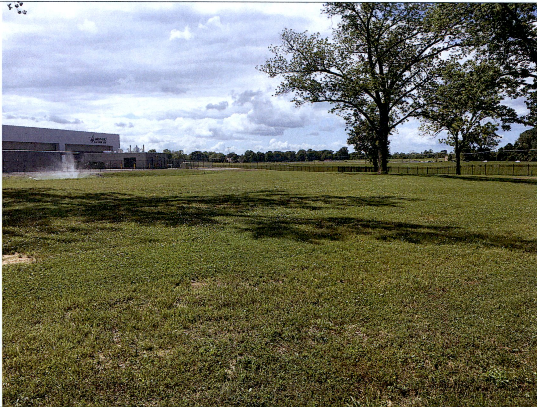
Area around Fire Water Ponds looking back toward Hangar 14.
